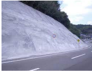
公路边坡检测 Roadside slope inspection
