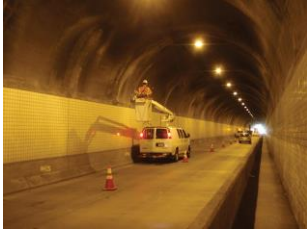
隧道检测 Tunnel inspection
